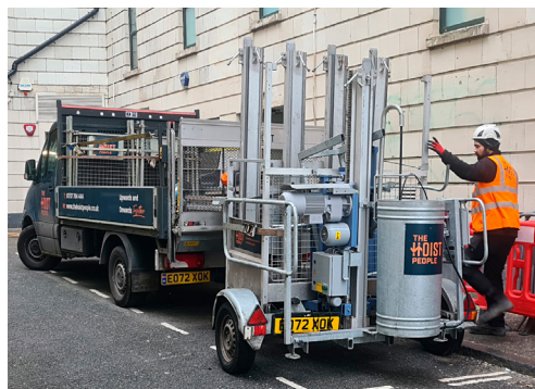
Towed to the site by trailer
