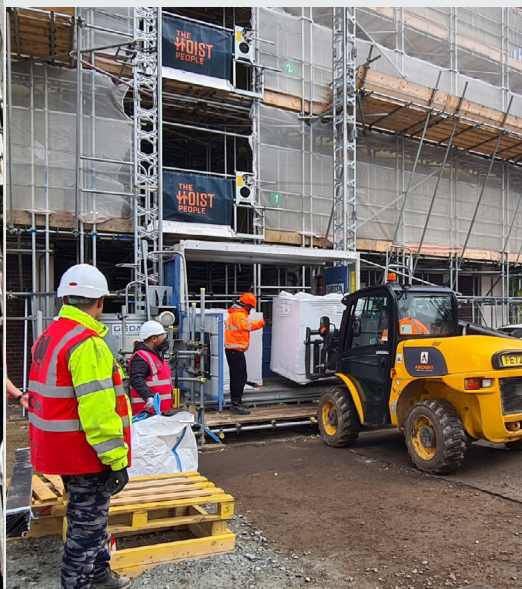
Loading the hoist at the base position
