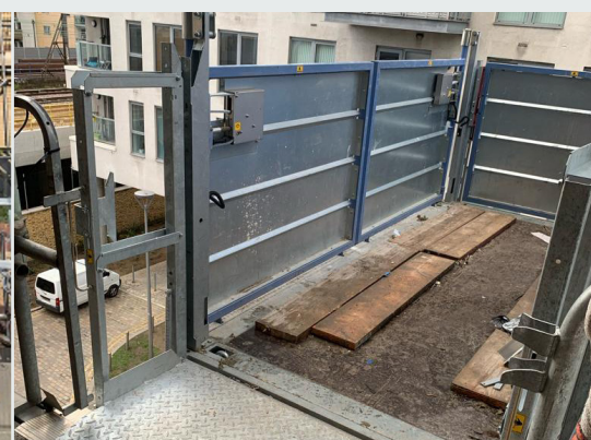
Hoist at the landing position
