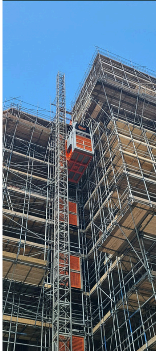
Hoist at the base position
