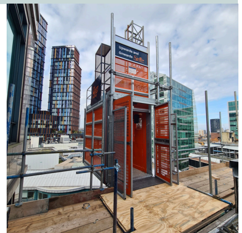
Hoist at the landing position
